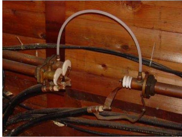
Figure 14.52: Flexible coaxial cables connected to rigid lines.
